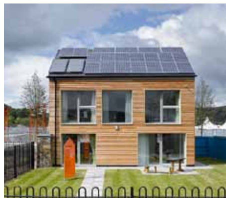
Larch House Ebbw Vale - South Facing
