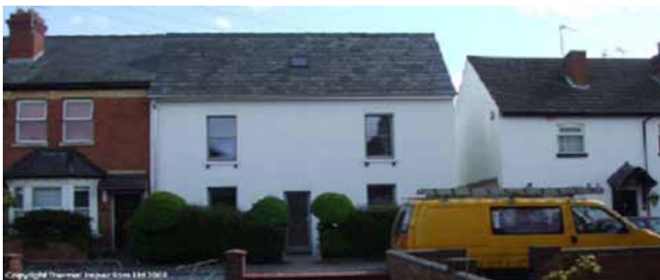
Simmonds.Mills / Thermal Inspections Ltd
